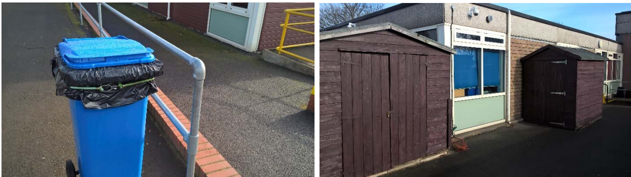
View of the waste bins and wooden sheds
