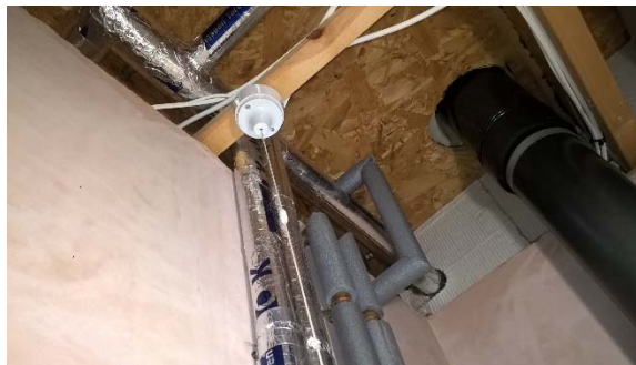
View of the boiler room ceiling in Building 3
